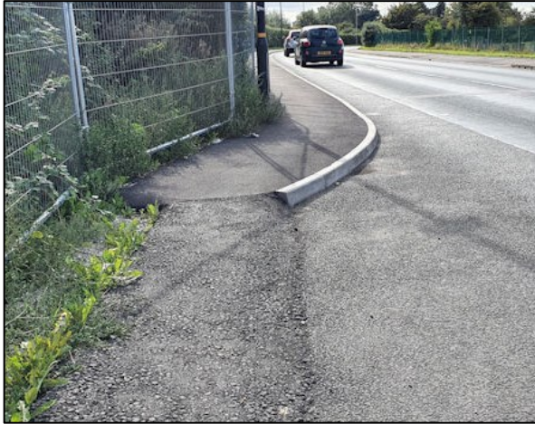
Photo 3.1-1: Western most radius section of unfinished bell mouth
